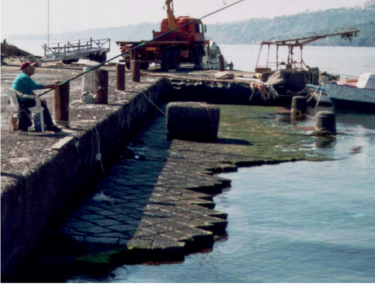
Fig. 6. Old and new docks in the Stazzo port during ebb tide.
