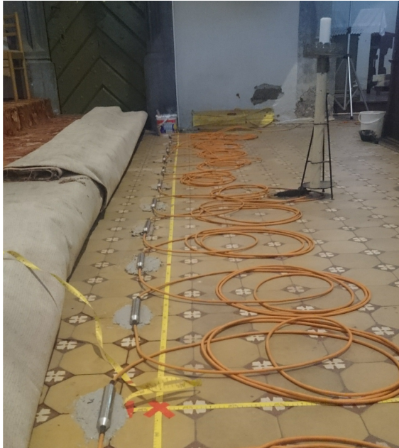
Fig. 4. Installation of the ERT electrodes section along a line inside the church of St. Catherine in Banská Štiavnica. Grounding conditions between the electrodes and the floor were improved by a bentonite bed (for every single electrode outlet).
